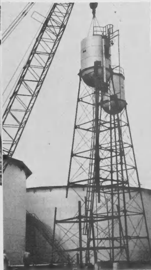
WHILE THE tall crane held the tank from above, the supporting legs were progressively cut off from below. As the legs were shortened the tank was lowered until at last it rested close to the ground where it was of such size that it could handily be placed on a truck and carted away as scrap.
